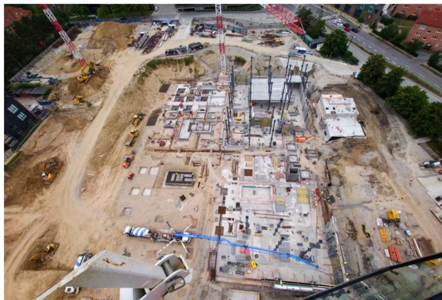
Construction Zones 1 & 2 overall view
