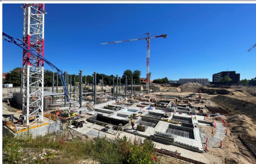
Construction Zones 1 & 2 overview
