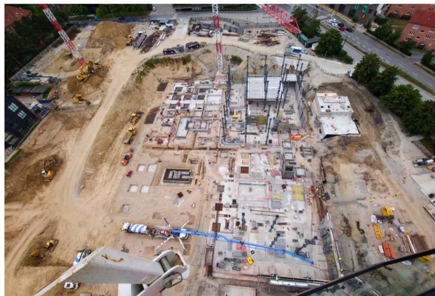
Construction Zones 1 & 2 overall view
