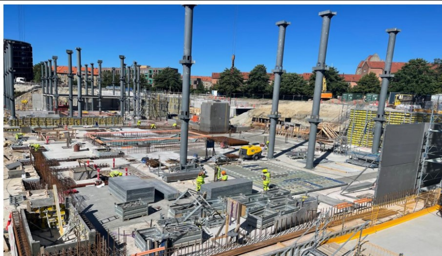
Construction zone CZ1.3 overview
