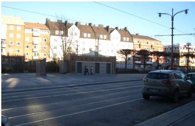
Omformerstation i Stockholm
